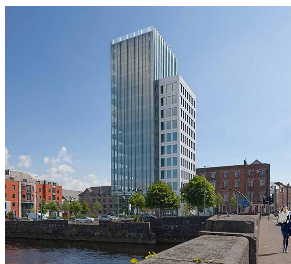
Approved Landmark Building at Bank Place
