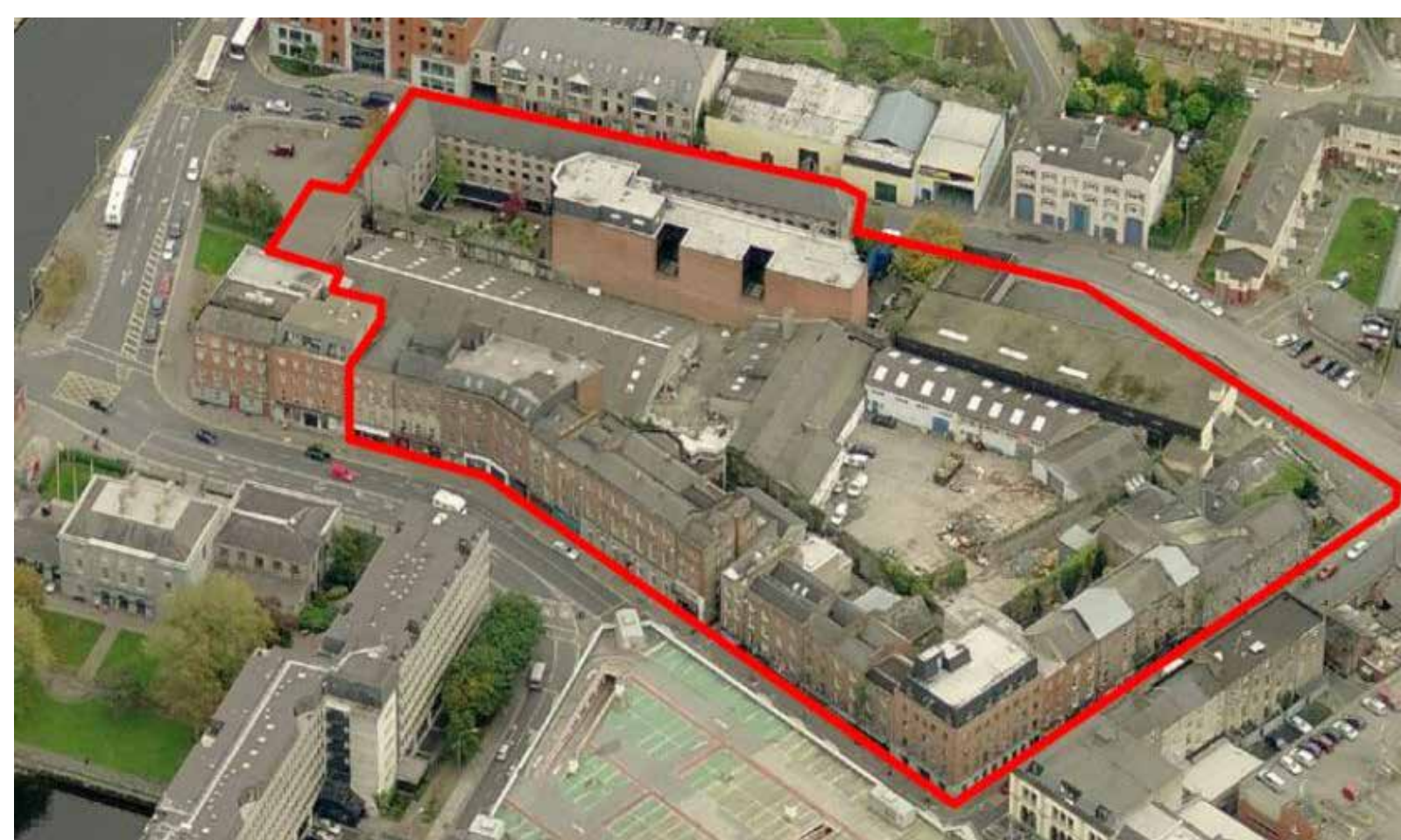
Site prior to demolition
